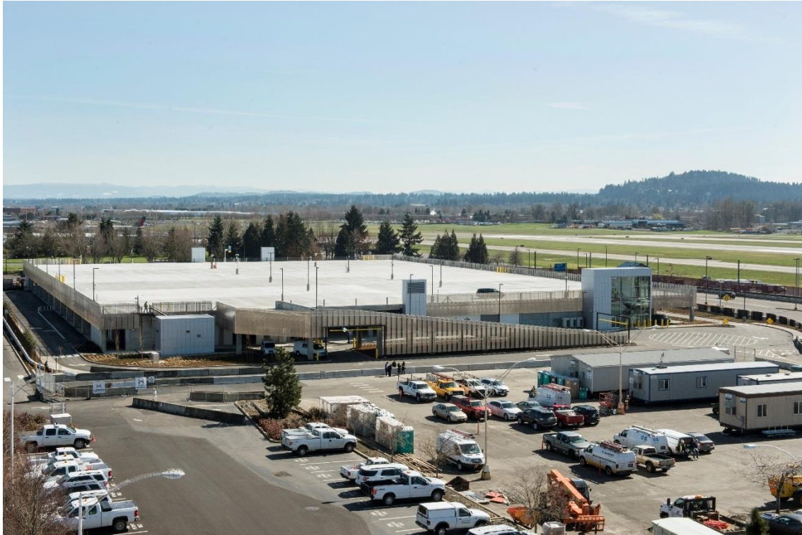
The Portland International Airport Quick Turnaround facility.
