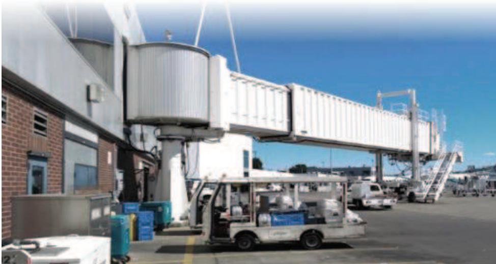
All but four of the PBBs at PDX were manufactured by JBT AeroTech. Mitsubishi, which no longer produces PBBs, manufactured the PBBs at Gates B1, B2, B3 and D2. The Gate B1, B2, and B3 PBBs were installed in 1986, and the Gate D2 PBB was installed in 1985. PBBs generally have a 30-year life expectancy.
