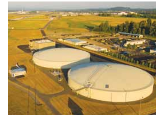
Storage tanks are part of PDX's enhanced deicing treatment system.
