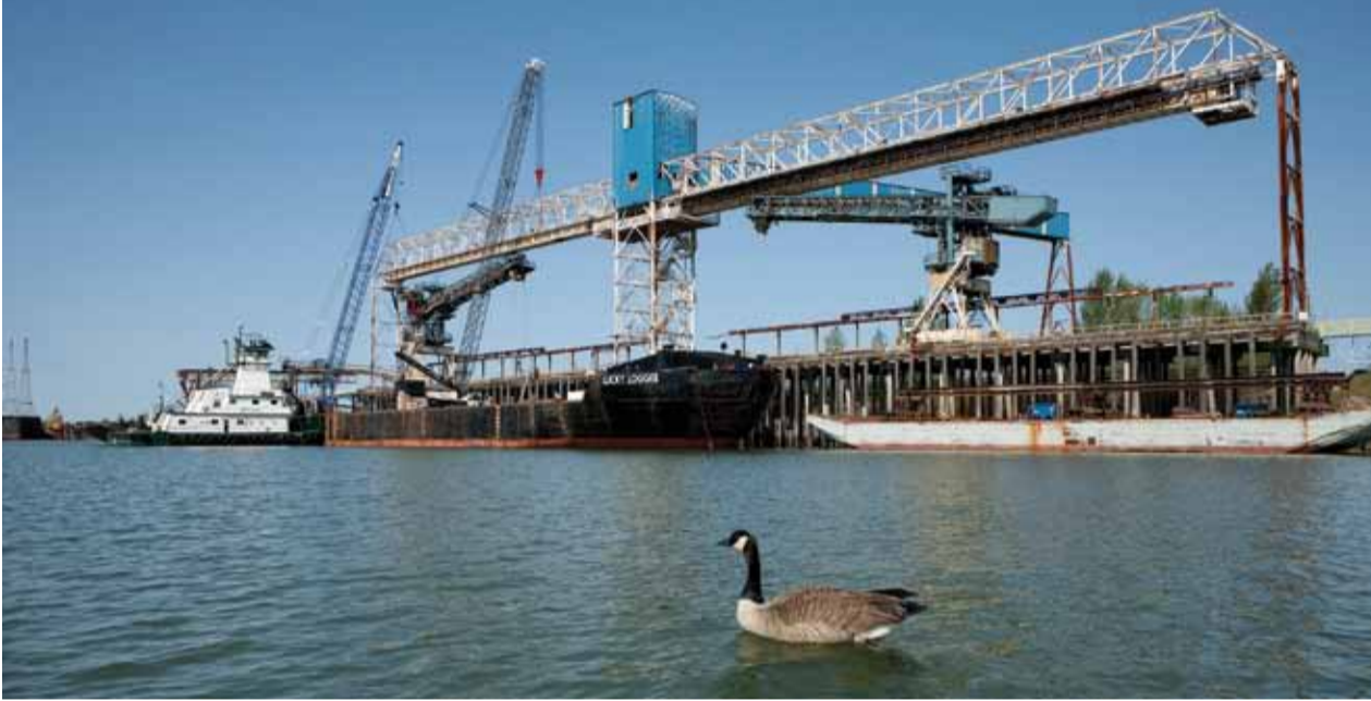
Out with the old; in with the new: Removal of outmoded grain conveyances makes way for a new pipeline rack system.
