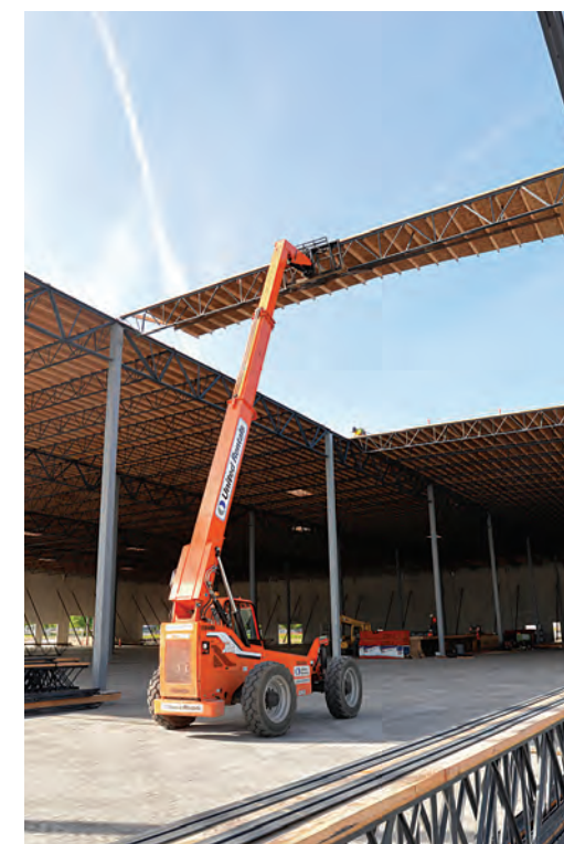
PDX Logistics Center under construction
