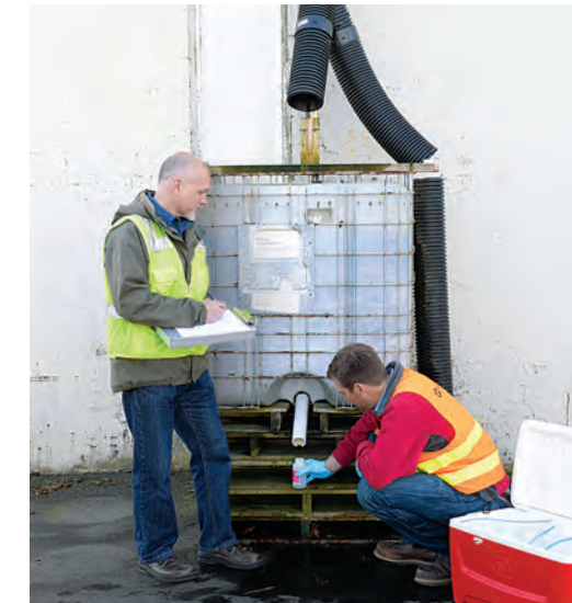
New Portable Media Filters treat stormwater runoff.
