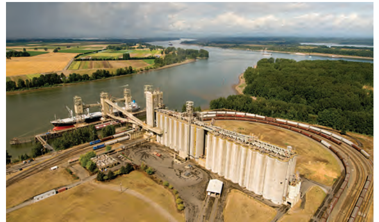
Columbia Grain, located near the confluence of the Columbia and Willamette rivers.
