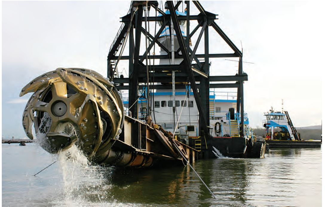
Dredging the navigation channel ensures Portland's role as an international trade gateway.
